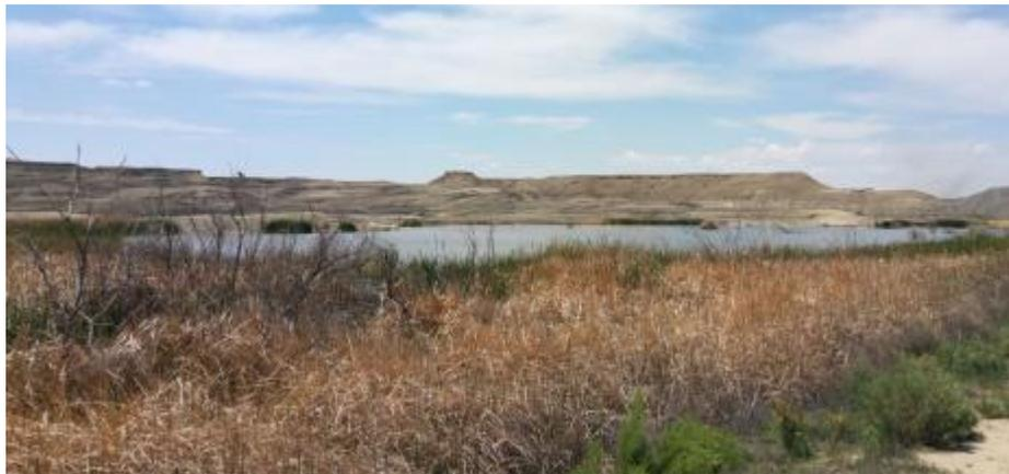
Navajo Mine environmental engineers used fluvial geomorphic principles to replace an inefficient diversion channel with a naturally functioning stream channel and stable landform. Using this method, Navajo Mine reclamation crews have created a landscape that is self-sustaining, able to withstand erosion and that provides natural wildlife habitat.
